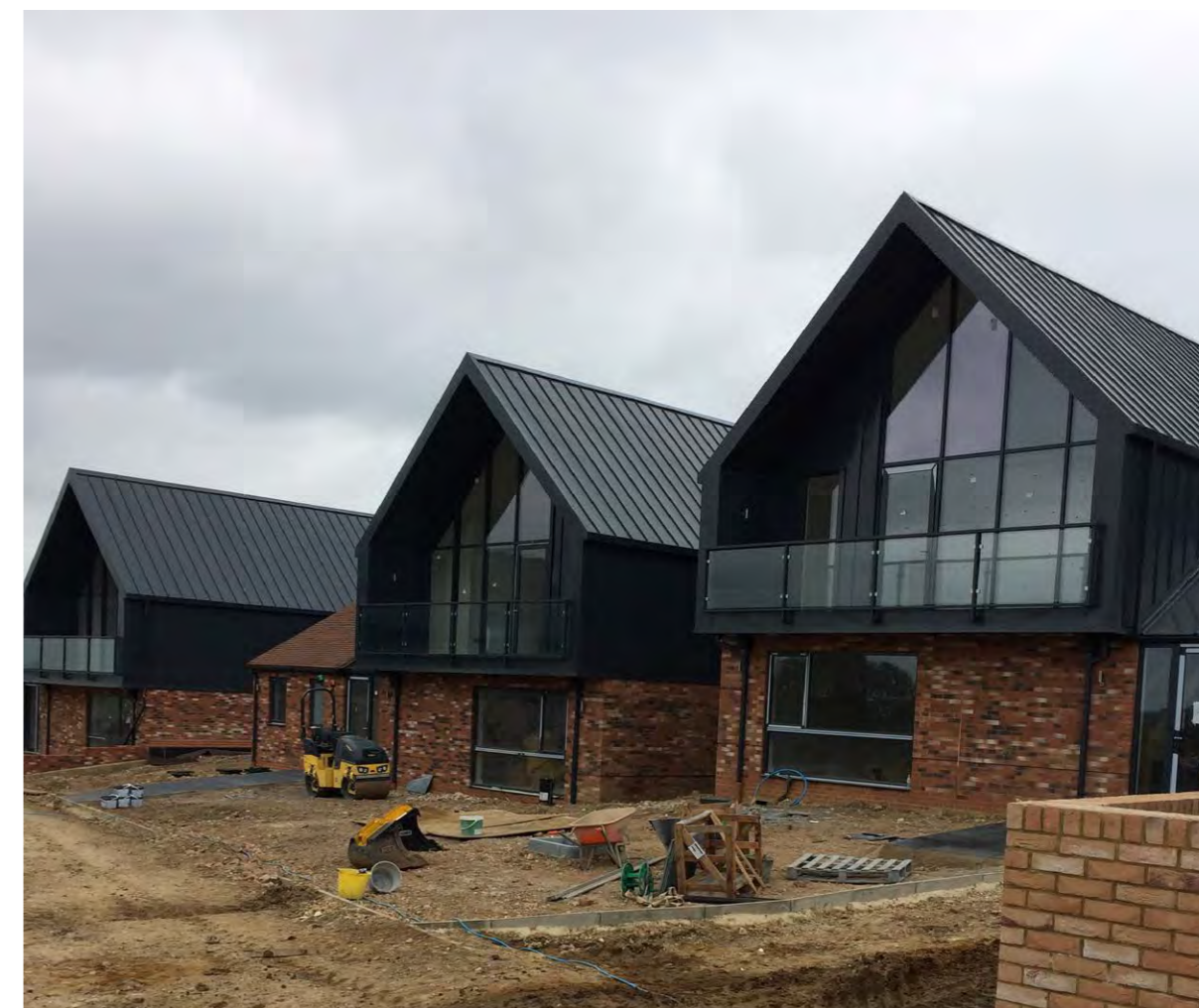
Figure 298: Plots under construction at Houghton Conquest
